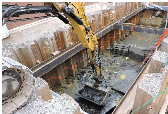
Figure 1: Remedial Activities at Mallinckrodt Plant 2 North
